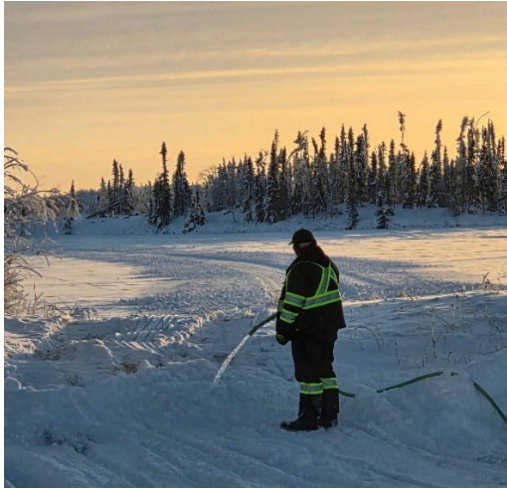
Building a ramp. Photo credit jvtcwinterroad.ca
